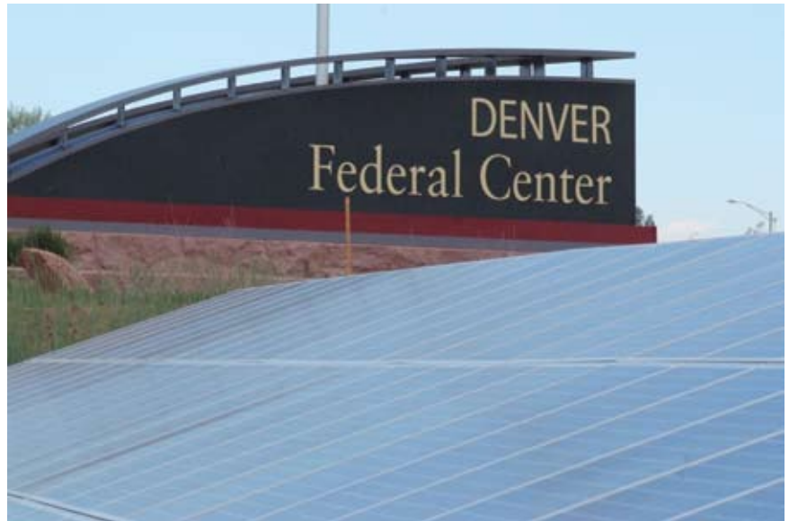
The Denver Federal Center will install roof-mounted solar panels that will save over $300,000 in electricity per year.
